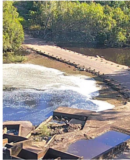
Teddington Weir floodway
