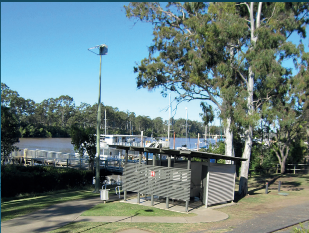
Portside Flood Monitor, Macalister Street, Maryborough
