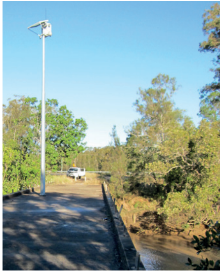
Saltwater Creek Bridge
