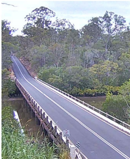
Burum River Bridge
