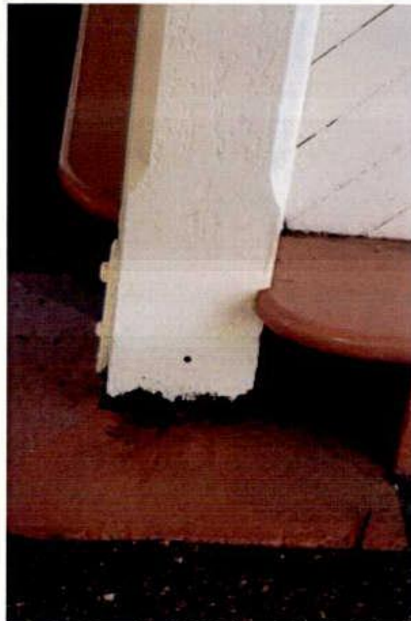
11 Detail view of a post supporting the fleche (tower) above.
