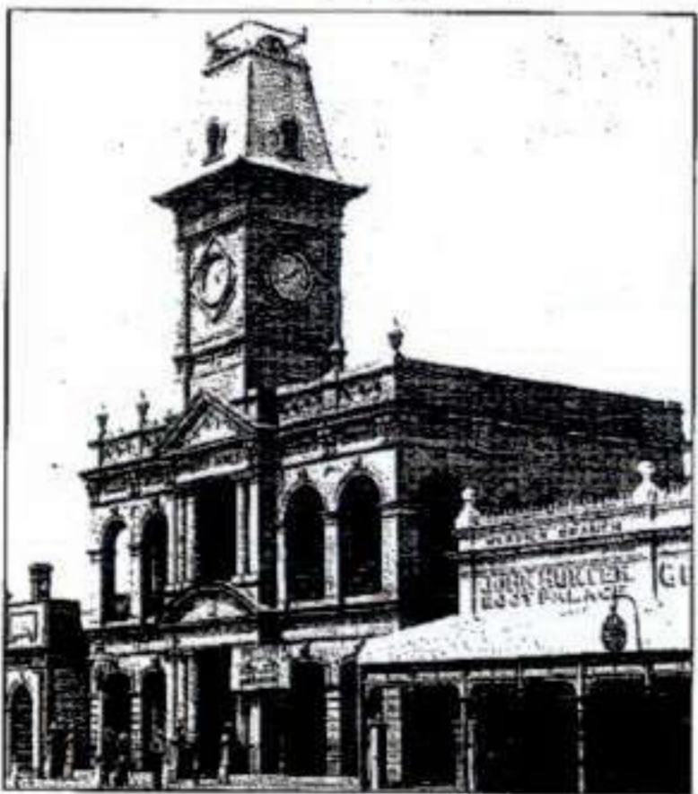
1885-88 Town Hall, Palmerin St, Warwick
