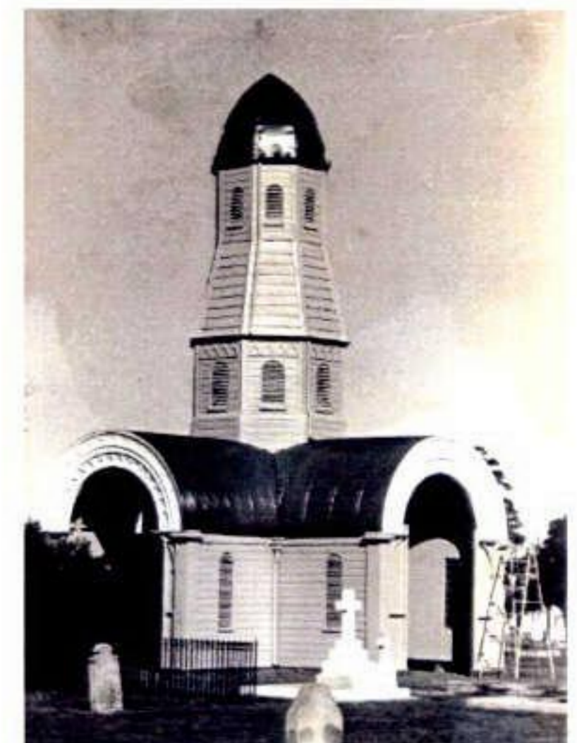
Figure 22. Mortuary Chapel 1983 after works completed. (Fraser Coast Regional Council)
