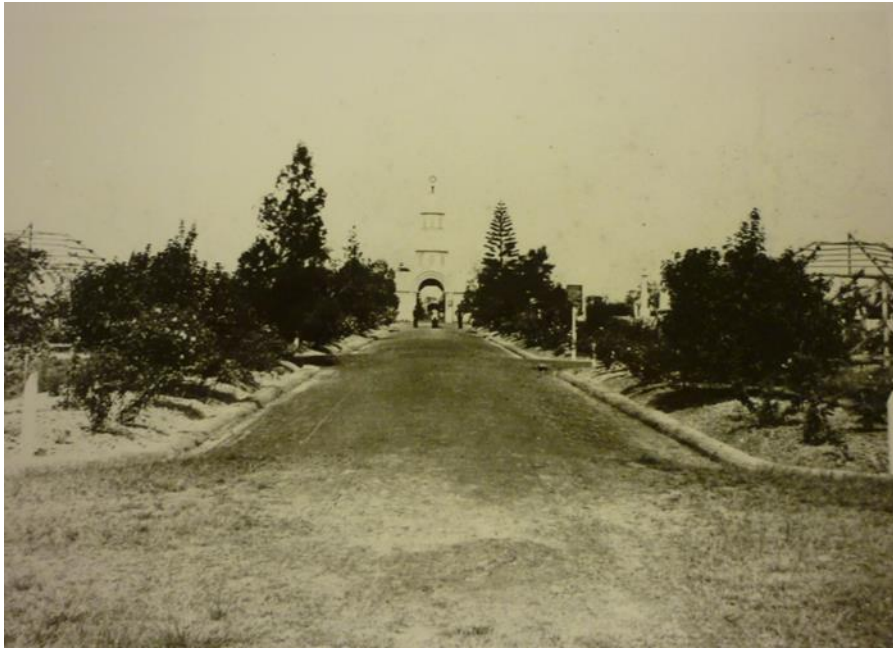
Figure 7: Example of kerbing and channelling, 1907. Note also the trellises to the left and right of the image. (JOL 76-7-8)
