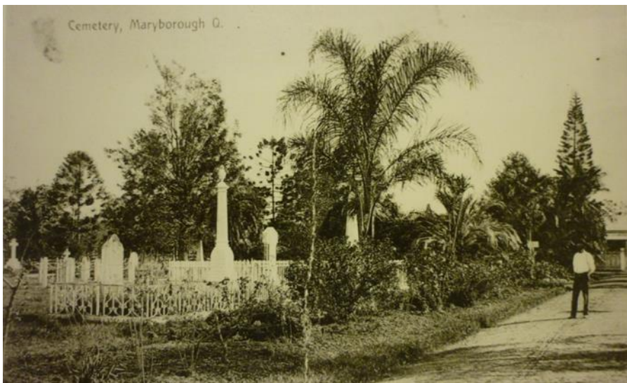
Figure 8: Photo dated 1911 showing the view to the Walker Street entrance. (JOL D10-5-90).
