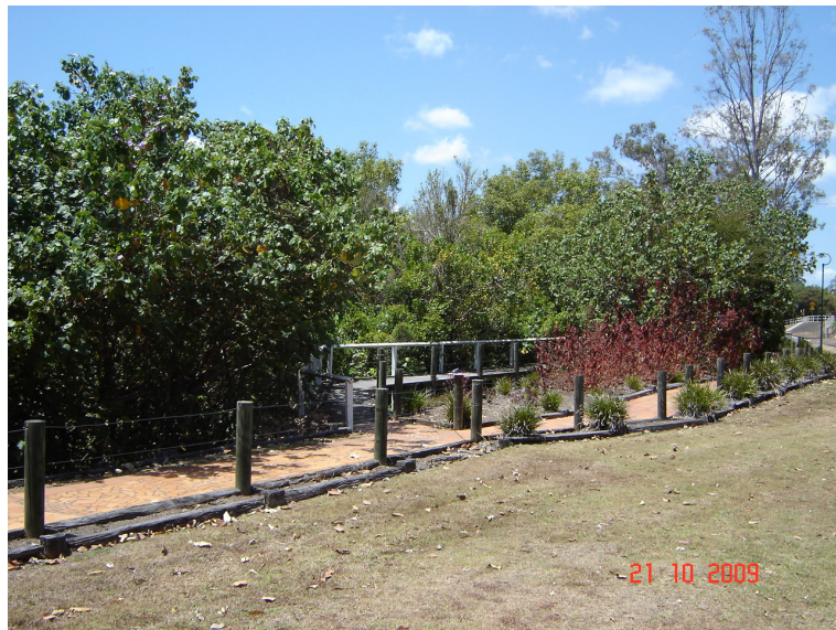
6 470458E 7175450N Downstream end of boardwalk (RBU3)
