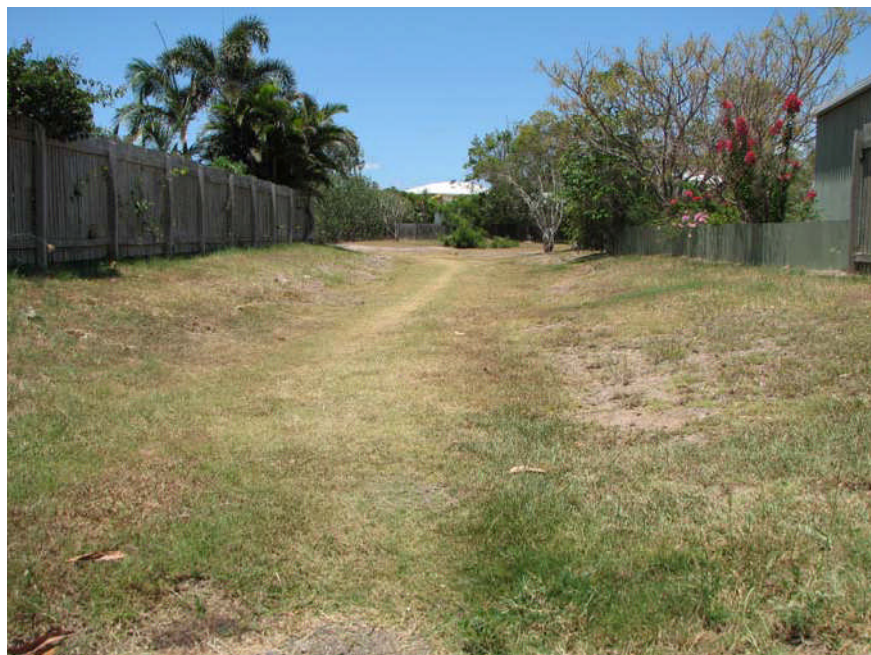
Photo 4: Downstream of Limpus Street outlet
