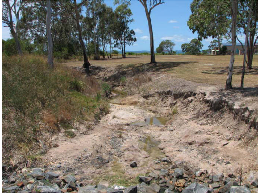
Photo 1: Downstream of Pulgul Street Culverts
