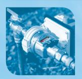
Your meter is a low metal pipe structure with a tap handle at one end and a meter dial at the other. It is usually located near your property's front boundary; normally at the centre, far left or far right side. Some are below ground level.
