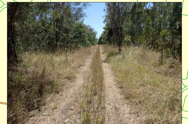
The corridor between Churchill Mine Rd and Colton is easily ridden and walked in its current condition. Unfortunately it is located within a mining lease.
