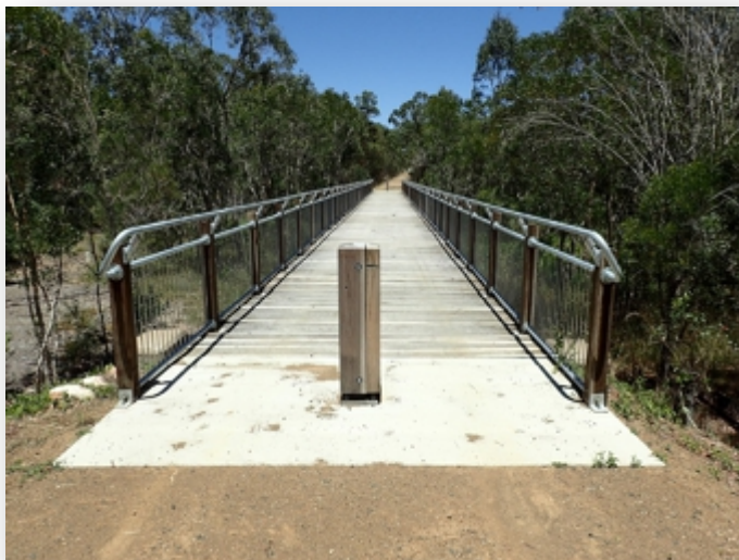
One of the old railway bridges refurbished for cyclist and pedestrian use of the recently constructed rail trail east of Dundowran Road.
