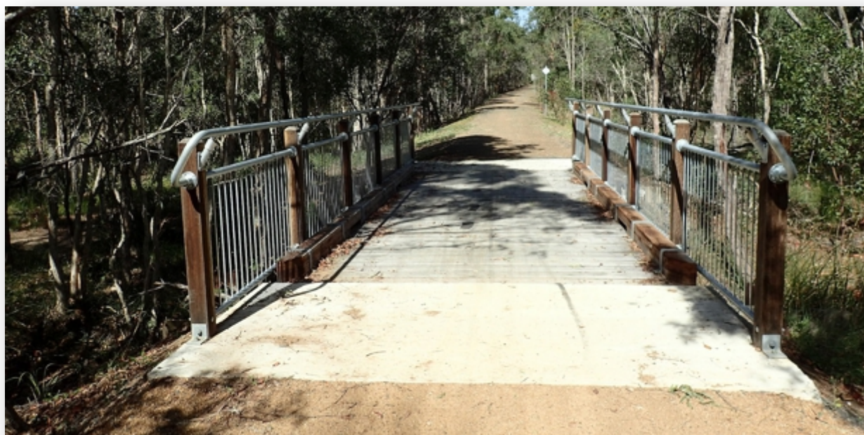
A compacted gravel surface and refurbished bridges (with solid timber decking and handrails) are features of the newly constructed rail trail between Piggford Lane and Dundowran Road.
