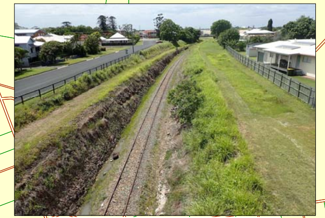
Looking SE down onto the railway corridor from the pedestrian bridge at Tooley St.
