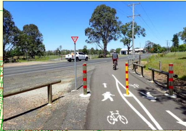
This design at Chapel Rd at Nikenbah provides a safe at-grade road crossing for trail users.
