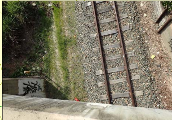
Minor deviations may be necessary where there is limited space between operating railway and abutments.
