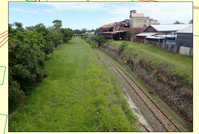
Looking NW down onto the railway corridor from the pedestrian bridge at Tooley St.
