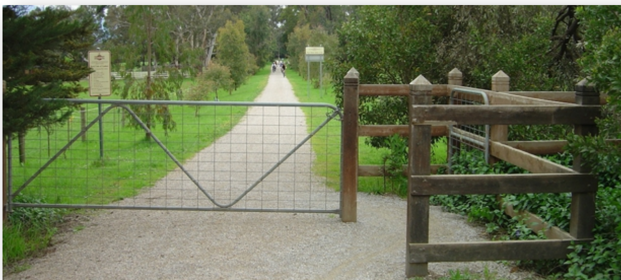
Above: the Lilydale Warburton Rail Trail in Victoria uses a gating system with chicanes to keep unauthorised users off the trail. These chicanes are being lengthened to permit longer bicycles (e.g. tandems and hand pedal bicycles). The existing barriers on the Mary to Bay Rail Trail will keep motor vehicles off the corridor but do little to deter trail bikes.
