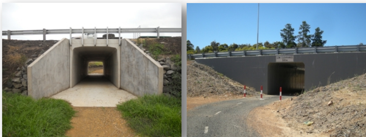
Above left: Port Fairy Warrnambool Rail Trail underpass of Princes Hwy in Victoria. Above right: Railway Reserves Heritage (Rail) Trail underpass of Great Eastern Highway near Clackline, WA.
