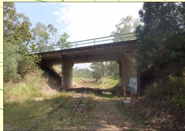
Space exists to route the rail trail in the underpass alongside the little used operating railway at Walker Rd.
