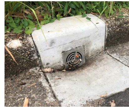
Figure 17: Batten Street, Kedron QLD. Street tree planting trial site for Water by Design's drainage system. Top Right: Drainage inlet. Bottom Left: Tree with drainage system installed. Bottom Right: Tree without drainage system installed.
