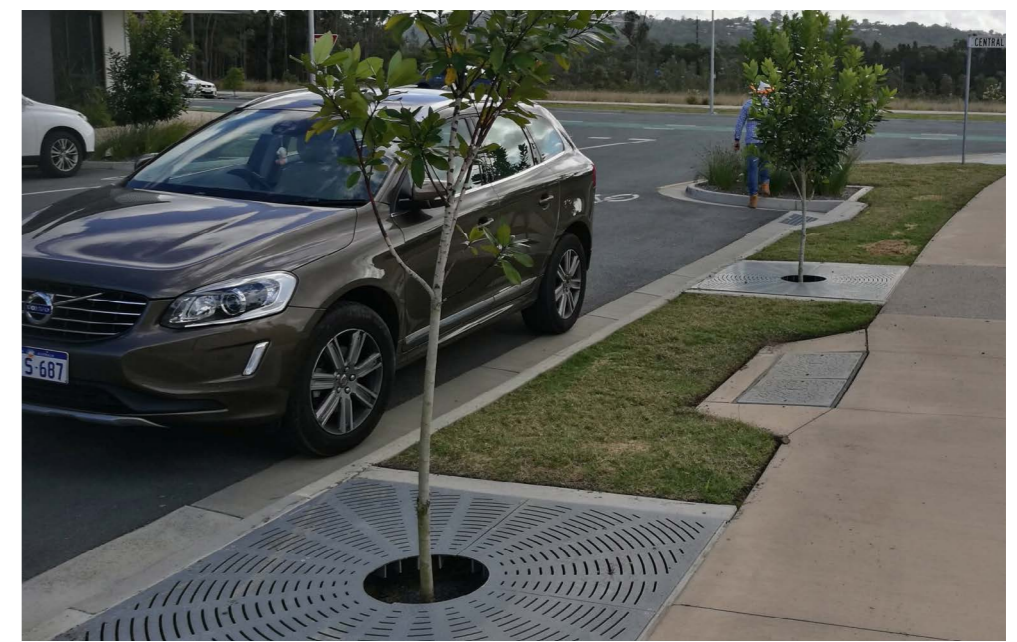
FIGURE 18 : Sippy Downs, Qld utilises bio-filtration tree pits within the verge to treat run-off.
