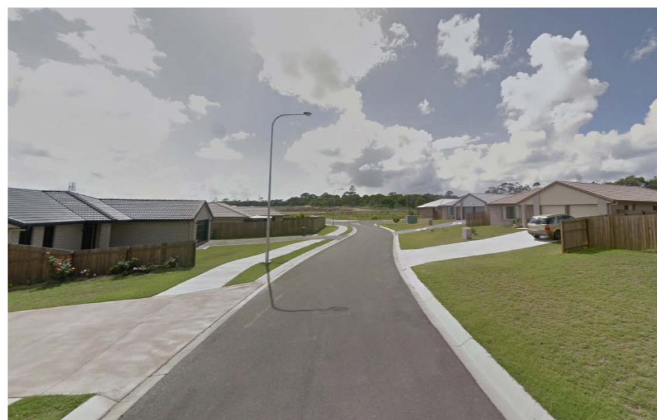
FIGURE 29b: Tasman Drive Street frontage shows garages within a 3-6m setback from front boundary.
