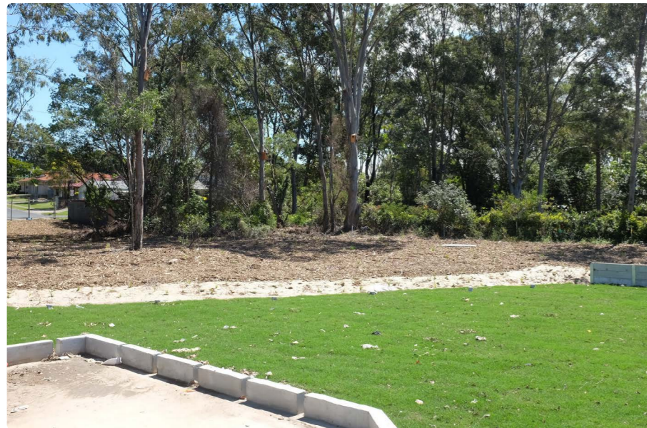
FIGURE 13 : Taigum, Qld has no trees installed within the bio-filtration device. This basin has temporary turf installed until the sediment risk from undeveloped lots is reduced.
