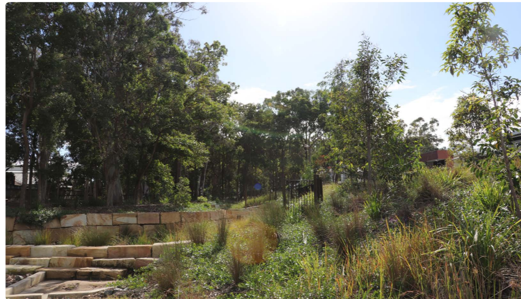
FIGURE 14 : Gumdale, Qld has trees installed within the bio-filtration device. Furthermore, with the consultation of an Arborist, the basin was designed to sit close to existing vegetation so the installation looks part of the natural landscape.
