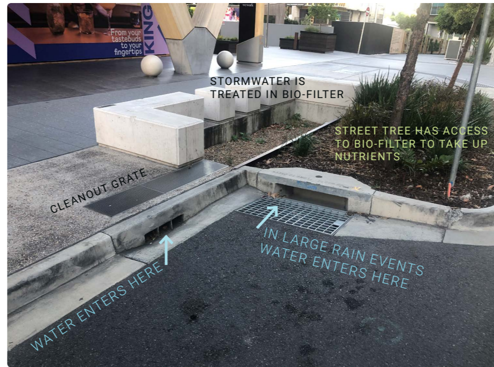
FIGURE 11 a & b : King Street, Fortitude Valley is an EDQ project utilising in street bio-filtration devices to treat surface stormwater. Co-located with street buildouts, this installation provides excellent tree growing potential. Bio-filtration areas are divided from pedestrian traffic by low walls that double as street furniture. This could be achieved also with standard street furniture, i.e. seats and bins..
