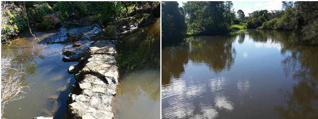
Figure 3-3 Waterbody C – a) Overflow weir, and b) Shallow waterbody upstream from the overflow weir.
