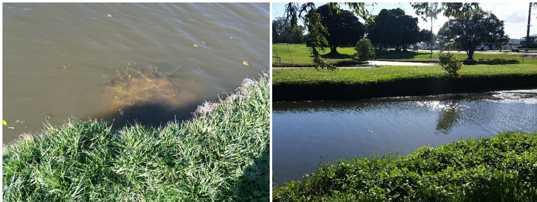
Figure 4-3 Localised edge erosion occurring adjacent to the golf course near the inlet to Ululah Lagoon.
