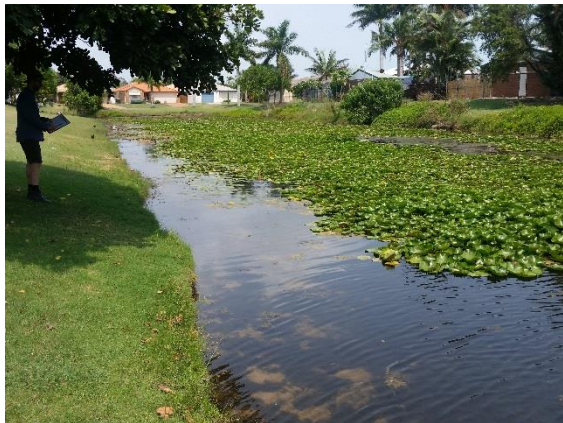
Figure 4-1 Minor scour present below grassed edges creating shallow vertical edge.
