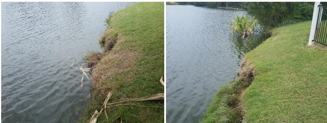
Figure 4-2 Eroded areas within Waterbody C: a) northern edge, and b) near Anembo Drive inlet.
