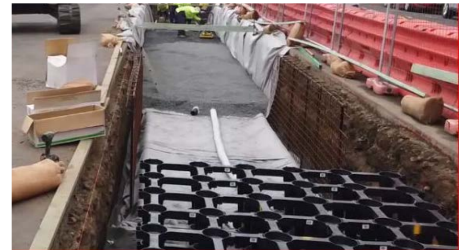
FIGURE 10 : StrataVault system tree trench installed in a roadway, Inverell, NSW 2018. Image courtesy of Citygreen.
