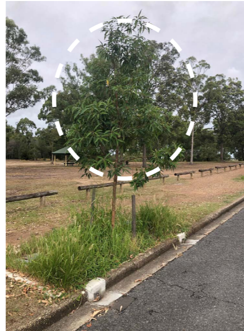
FIGURE 16: Detail for street tree Bio-filtration device from Water by Design where a simple kerb inlet and ag drain provides a water source for the street tree.
