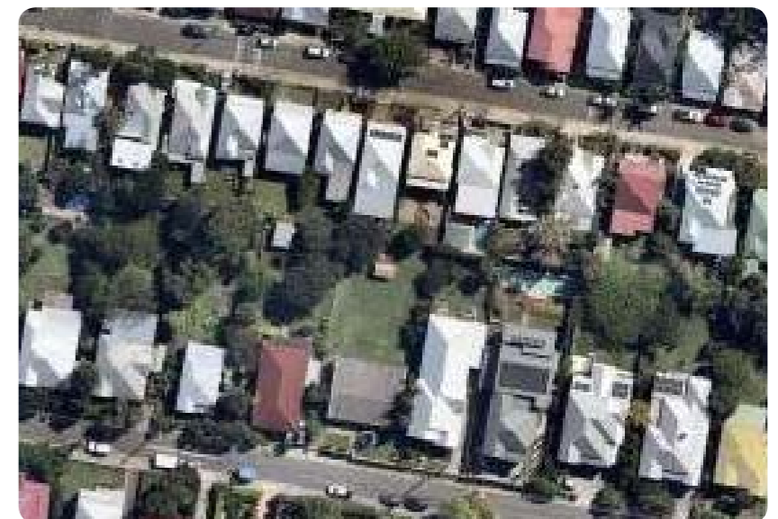
FIGURE 28a & b : New housing, as seen at Pialba 4655 (top) has slightly wider lots (15-20m wide) compared to older housing, West End 4101 (bottom) where lots are mostly 10m wide. New houses are also much larger than older two storey homes. Slab on ground design, being cheaper than two storey homes, means more rooms are spread across a larger footprint than multi-storey homes.
