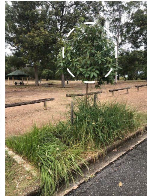
FIGURE 18 : Sippy Downs, Qld utilises bio-filtration tree pits within the verge to treat run-off.
