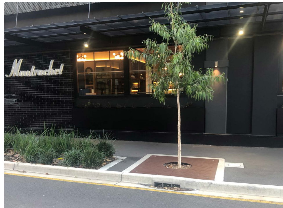
FIGURE 12 a & b : King Street, Fortitude Valley allows street trees to use low flow stormwater whereby water enters the tree pit from the curb. Higher flows mostly bypass directly to the curb inlets. Roof water from awnings can also pass through these devices although high flow bypass is required.
