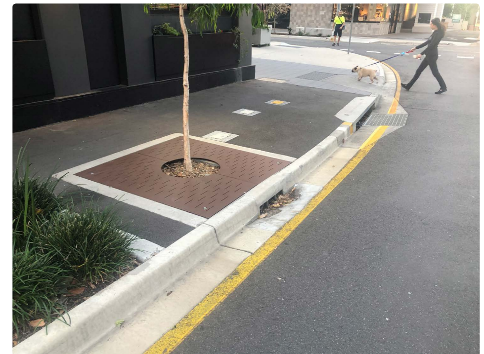
FIGURE 12 a & b : King Street, Fortitude Valley allows street trees to use low flow stormwater whereby water enters the tree pit from the curb. Higher flows mostly bypass directly to the curb inlets. Roof water from awnings can also pass through these devices although high flow bypass is required.
