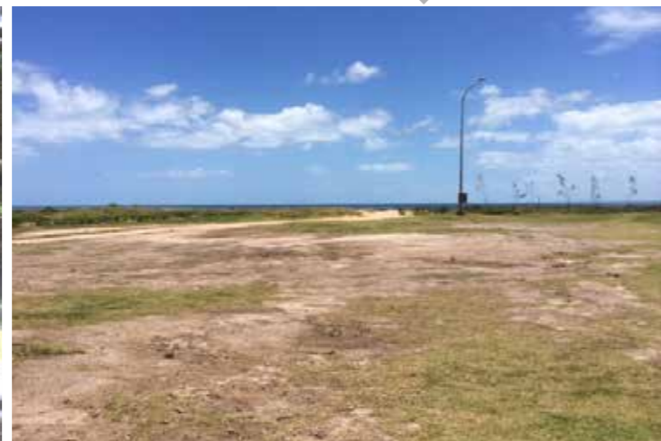
Drainage issues affecting open space
