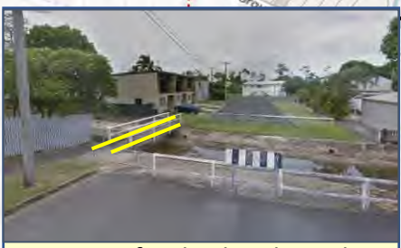
Existing footbridge through Toon Toon Creek (to provide pedestrian connectivity)
