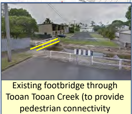
Existing footbridge through Toon Toon Creek (to provide pedestrian connectivity)
