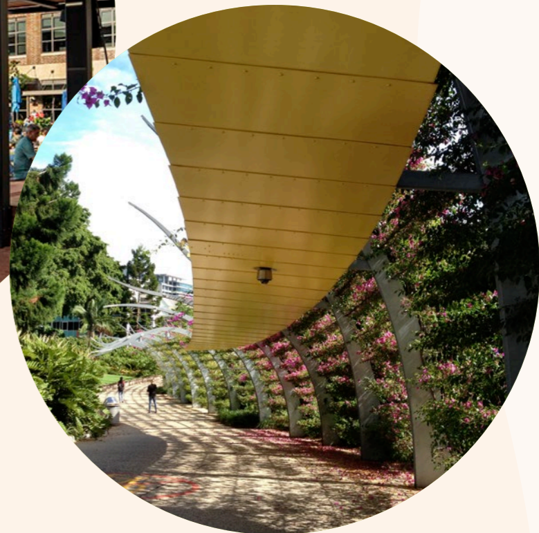
Right: Covered pathway with lighting for safe pedestrian and cyclists movement
