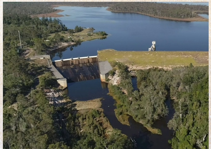
Aerial image of Lenthalls Dam and spillway.
