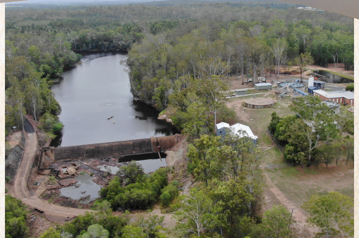
Aerial image of Teddington Water Treatment Plant and Teddington Weir.
