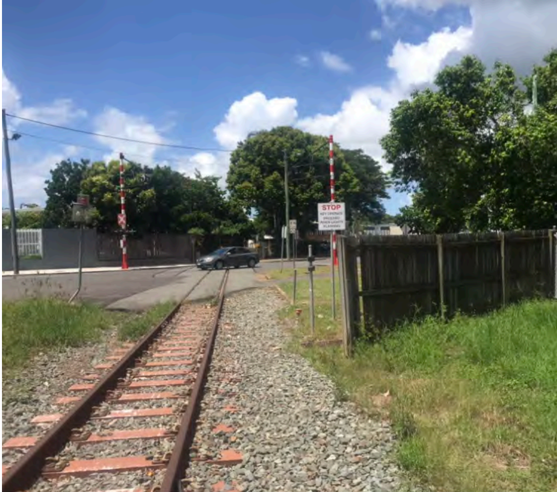
21. Kent Street crossing. Alan and June Brown RV park to the right.
