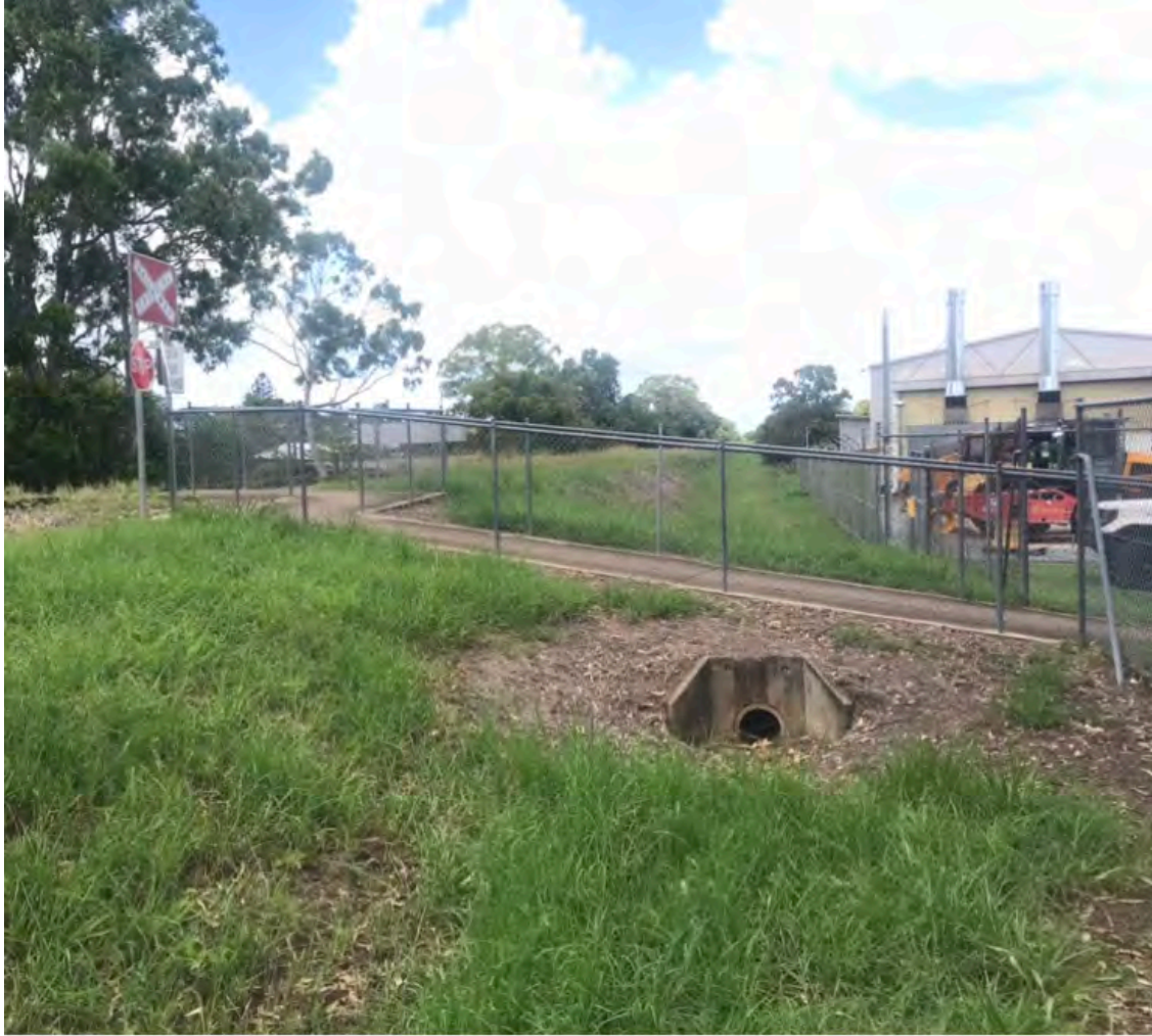
6. Morning Street pedestrian crossing approach.
