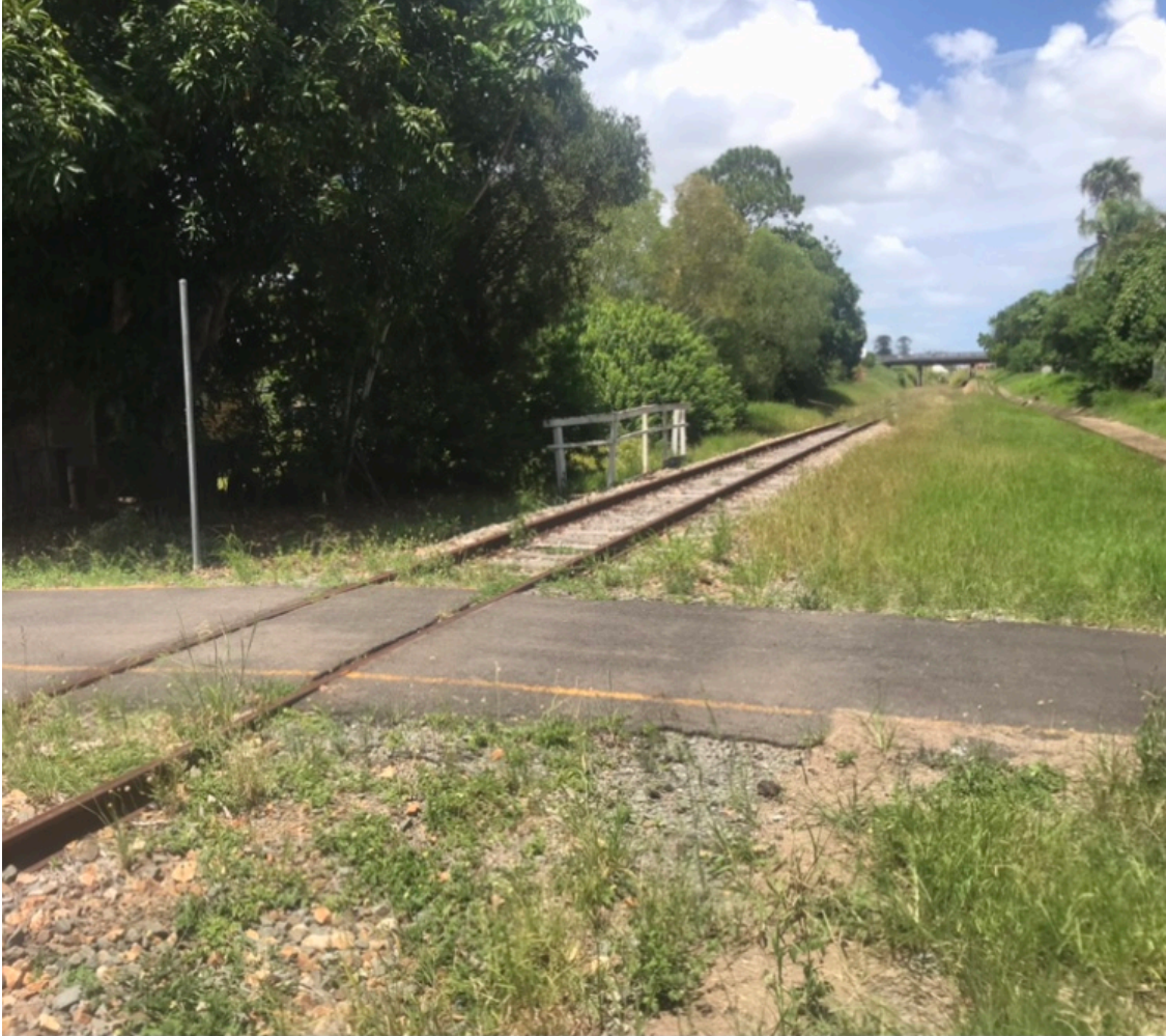
14. Cheapside Street pedestrian/cycle crossing.
