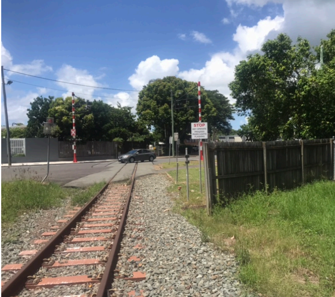
21. Kent Street crossing. Alan and June Brown RV park to the right.
