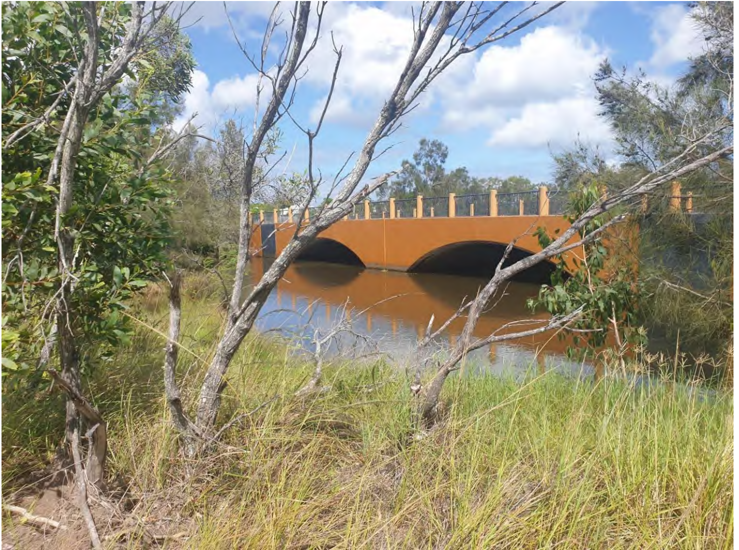
Figure 6-3 Endeavour Road Bridge
