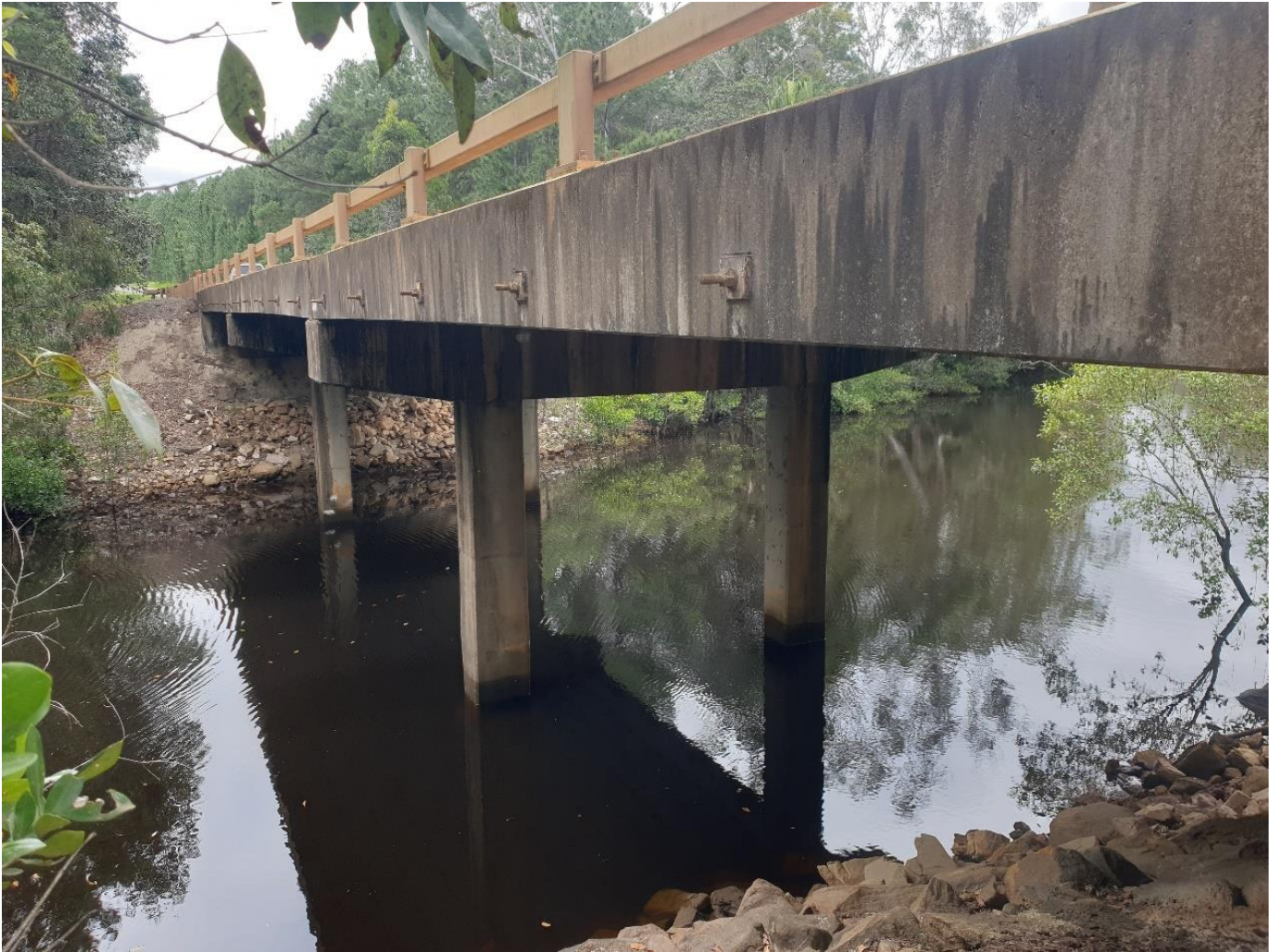
Figure 6-3 Big Tuan Creek Road Bridge
