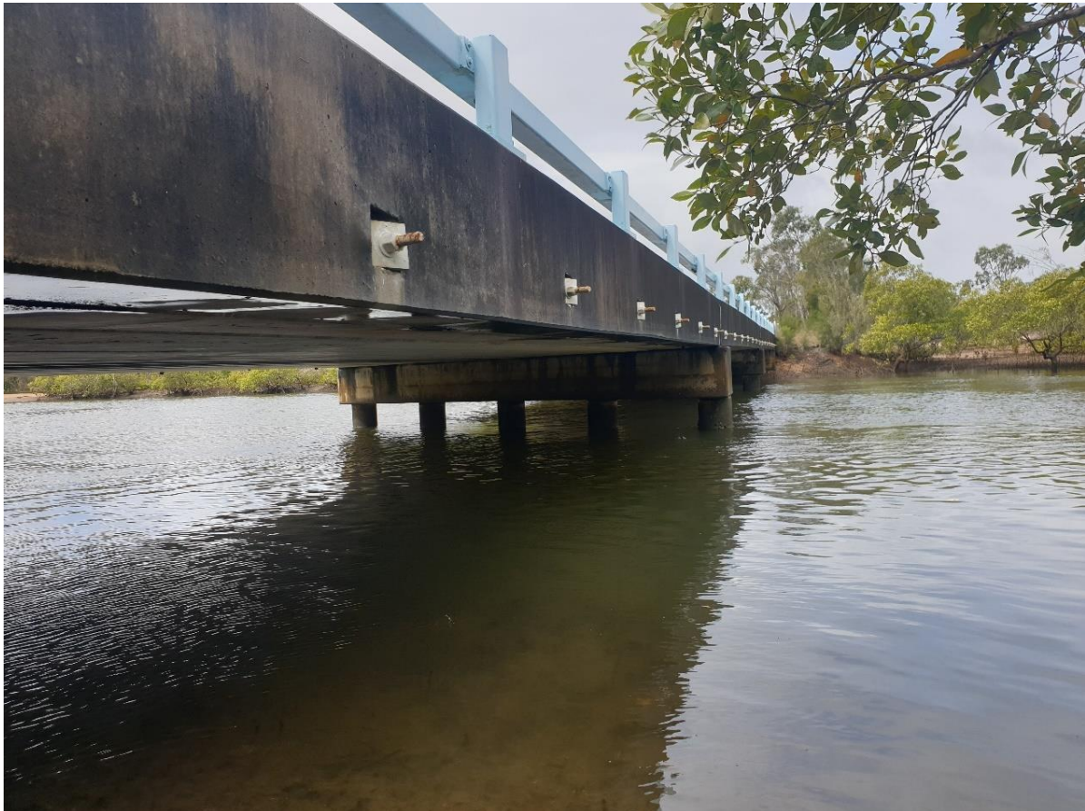
Figure 6-2 Wilkinson Road Bridge
