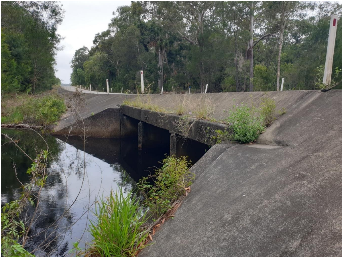
Figure 12-1 Scrubby Creek Causeway and Culverts
