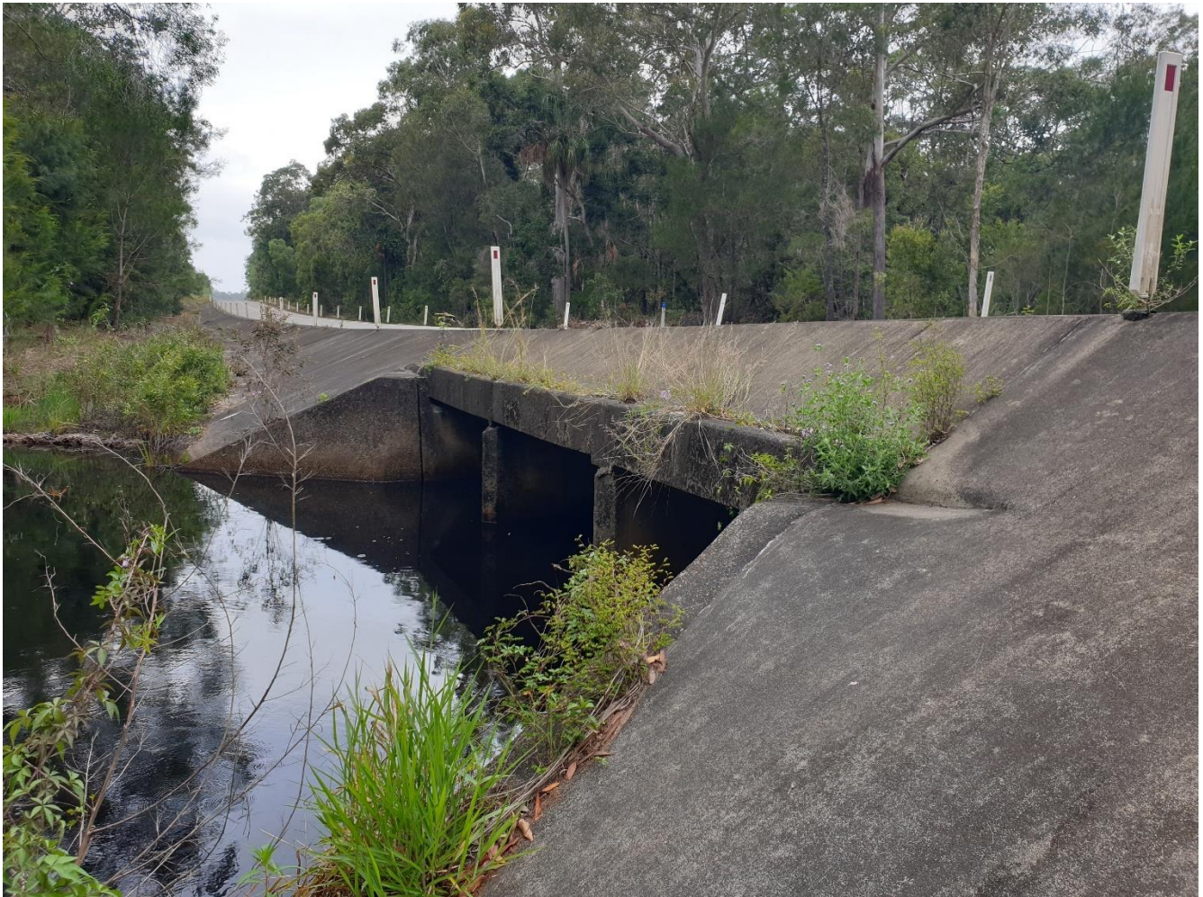
Figure 13-1 Scrubby Creek Causeway and Culverts
