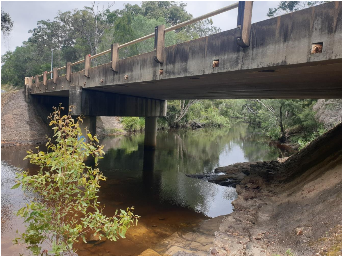
Figure 6-1 Poona Creek Bridge
