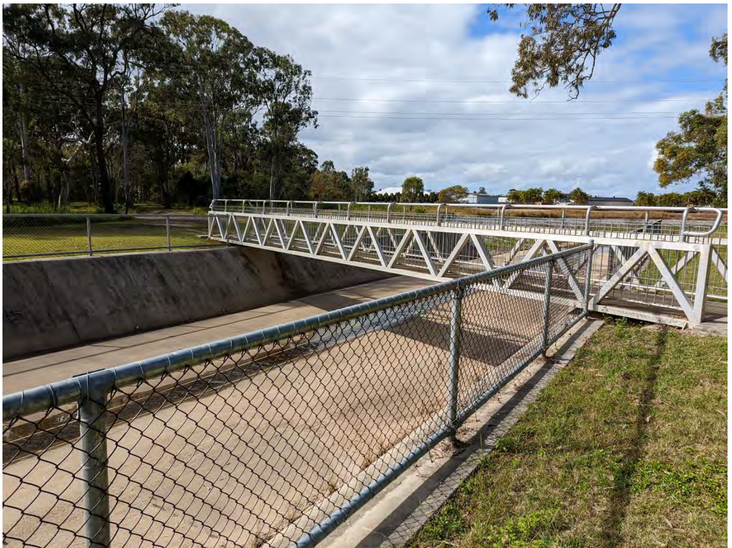
Figure 6-1 Doolong Road Pedestrian Bridge
