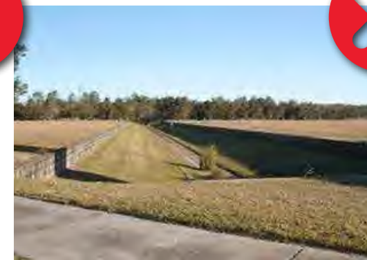
Hard-edged engineered drains - poor ecological function, often dependent on mowing to maintain conveyance capacity.
