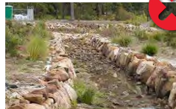
Rock lined trapezoidal channels - poor ecological function, prone to weed infestations, difficult to maintain without using herbicides in waterway
