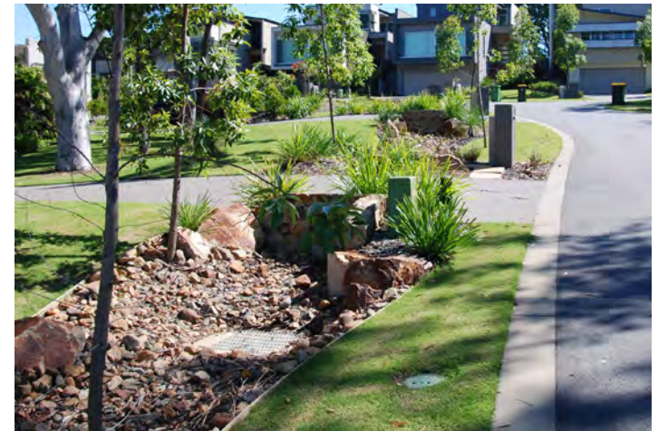
Flush kerb and one way cross fall elements of overall WSUD strategy
