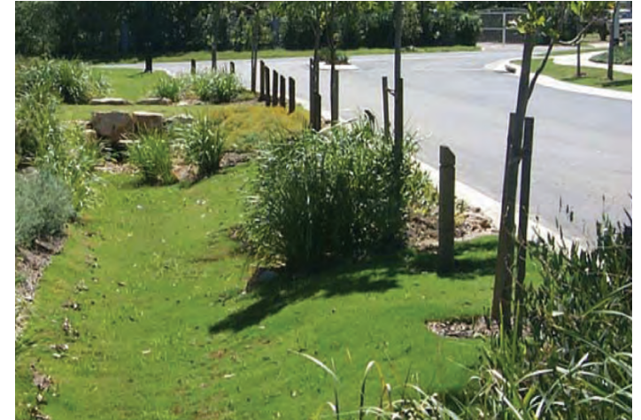
Road edge to parkland area
