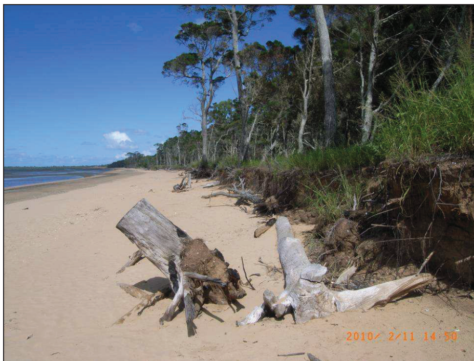
Plate 6: Erosion – Dundowran (approx. 1.4m high)
