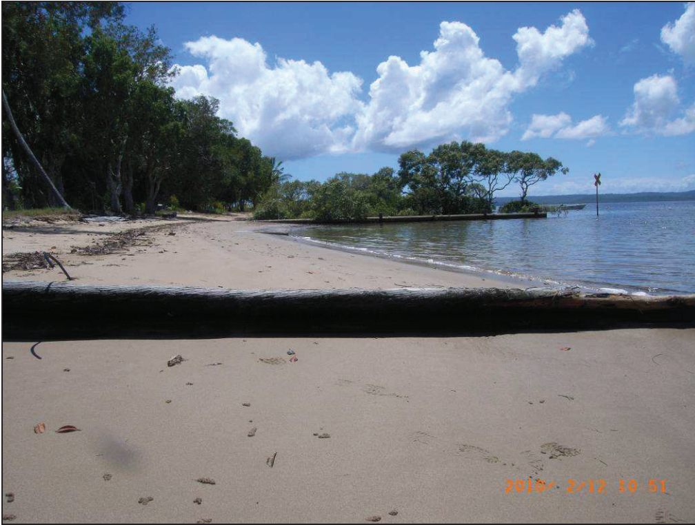
Plate 3: Stormwater Outlet: Poona
