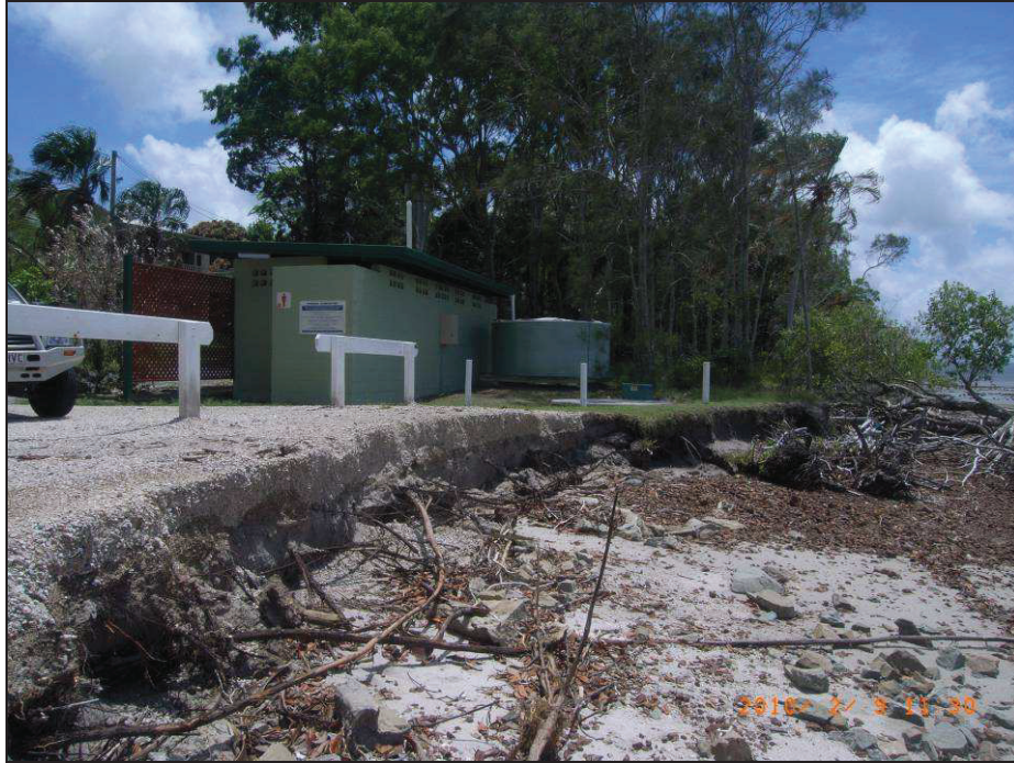
Plate 5: Erosion – Poona (approx. 1.0m high)
