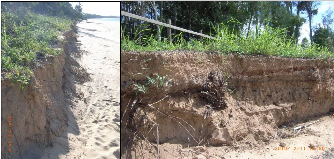
Figure 3.1: Erosion Scarp - Hervey Bay Area
