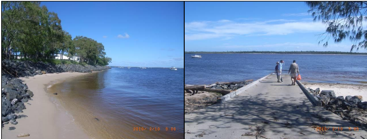
Figure 3.5: Existing Coastal Protection Works - Burrum Heads
