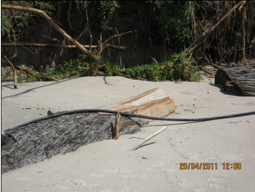
Figure 6.1: Exposed Telecommunications Cable
